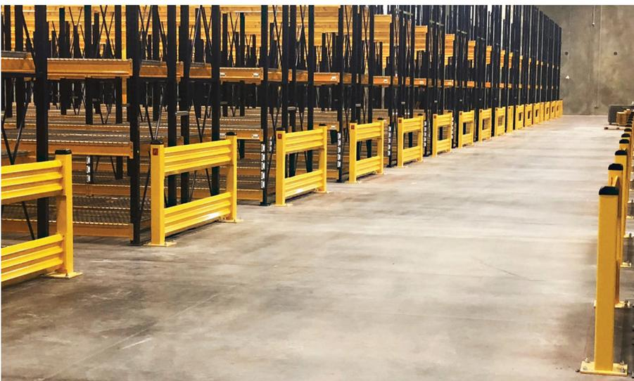
Strong end of aisle rack protection with offset baseplates
